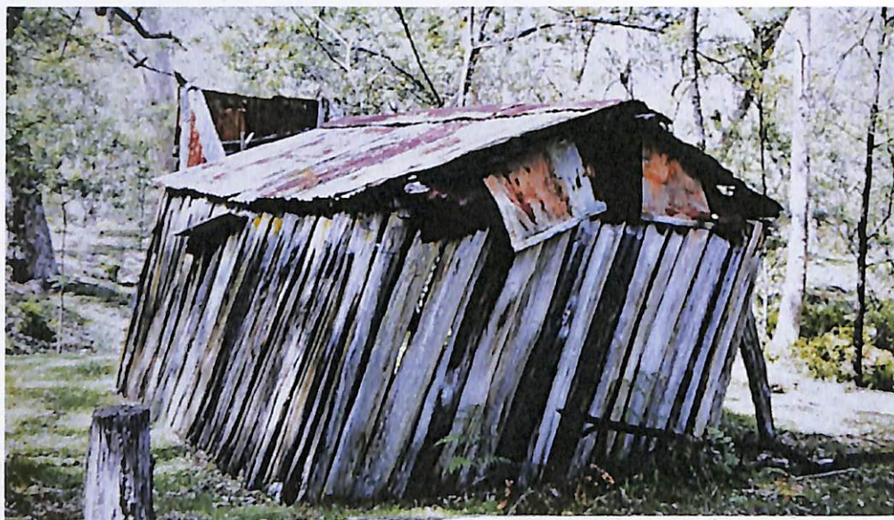
Figure 51: Super Sutherland's hut at Spring Mountain. Photo courtesy John Davidge
